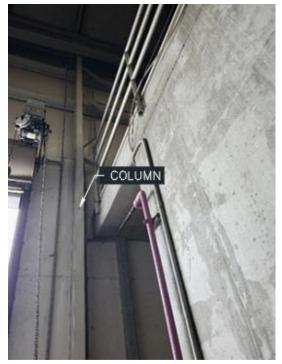
Picture 13: Concrete column pier
