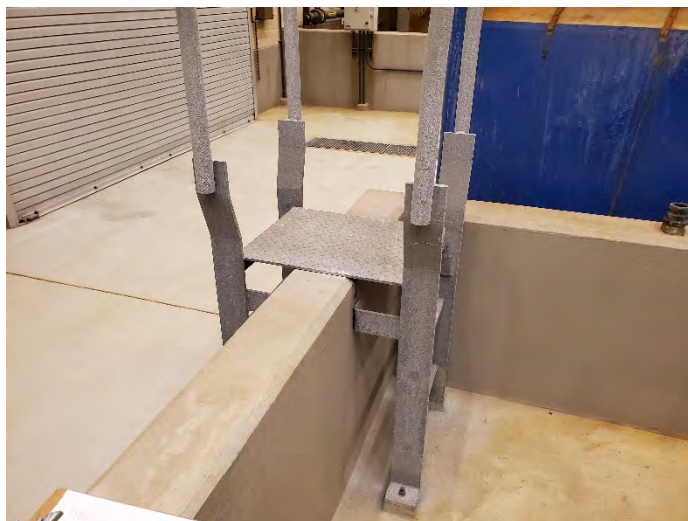
Figure 6 - Galvanized Access Ladder
