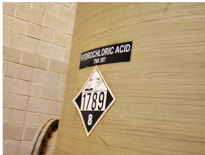
Figure 1 - Hydrochloric Acid Storage Tank
